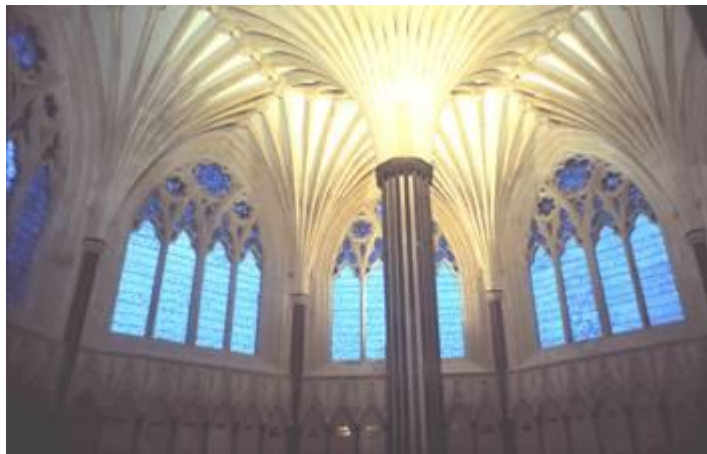
Figure 5. The Chapter House at Wells Cathedral, demonstrating the use of narrow beam tungsten halogen spotlights, from concealed locations.
