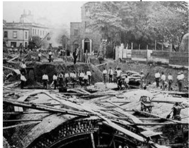
Fig.1 The chaos of the cut-and-cover method
