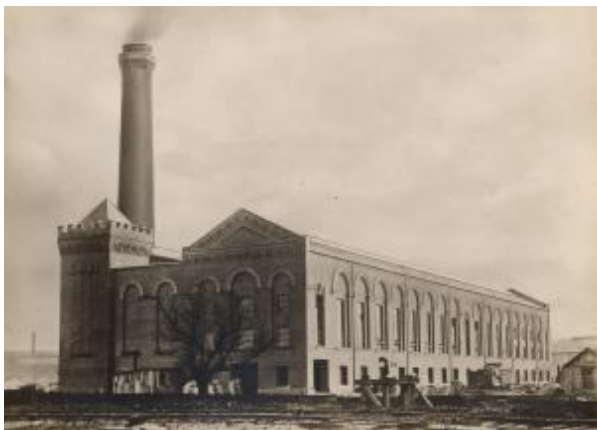
Fig.5 Neasden Power Station
