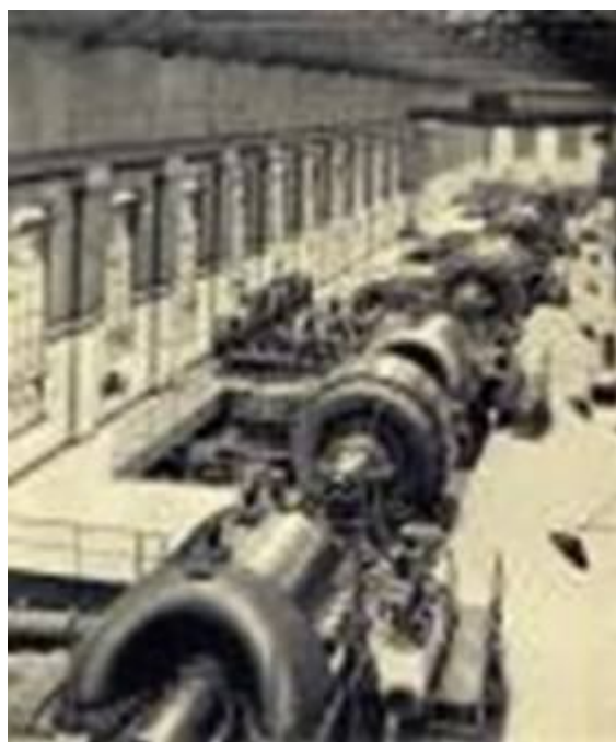
Fig.6 Neasden Station Plant
