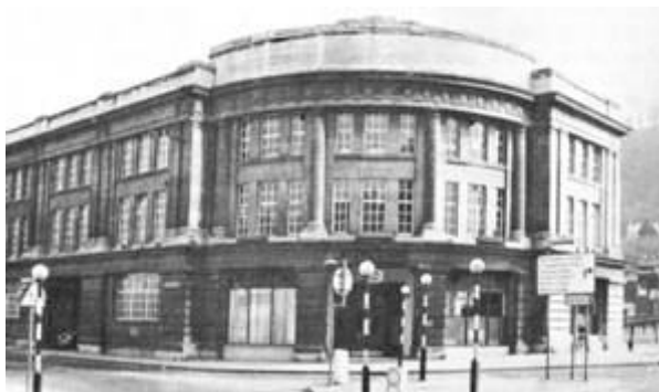
Fig.6 New Showrooms and Offices (Courtesy J. Roberts)
