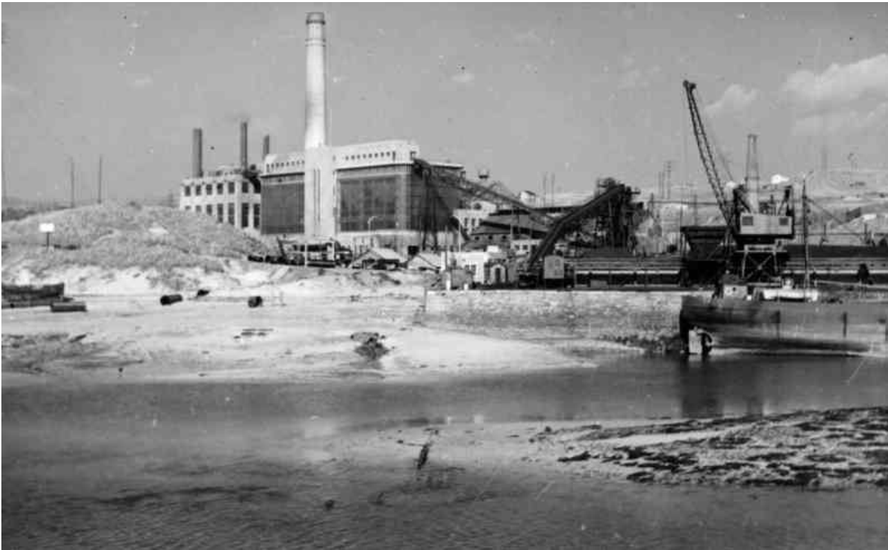
Fig4 Hayle Power Station circa 1950
