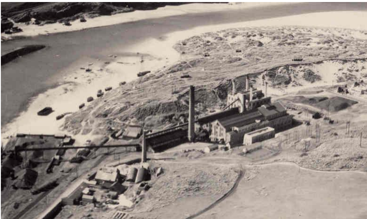
Fig. 2 Hayle Power Station 1934
