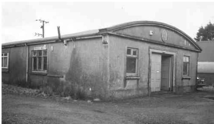
Fig.1 Princetown Generating Station Building
