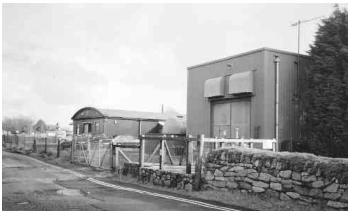
Fig.2 Old Generating Station alongside New One
